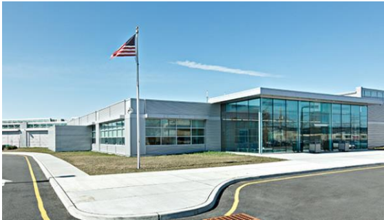
Bergen Co. Juvenile Detention Center, Teterboro, NJ Photo courtesy of Mast Construction Services website
