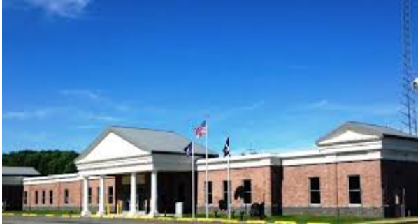
Delaware Co. Correctional Facility, Delhi, NY
