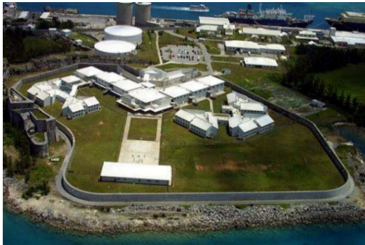
WESTGATE CORRECTIONAL FACILITY, BERMUDA.
