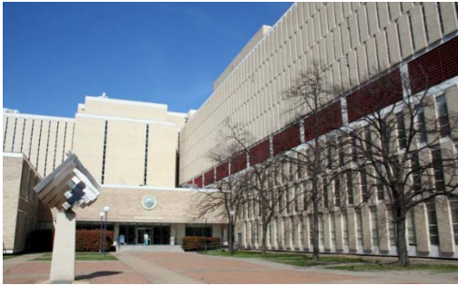
NORFOLK CITY PUBLIC SAFETY BUILDING
